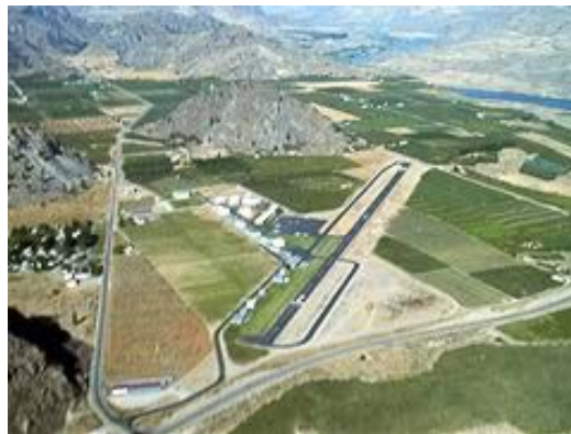
Expansion of the Chelan Airport is being considered in the revision to its comprehensive plan.
